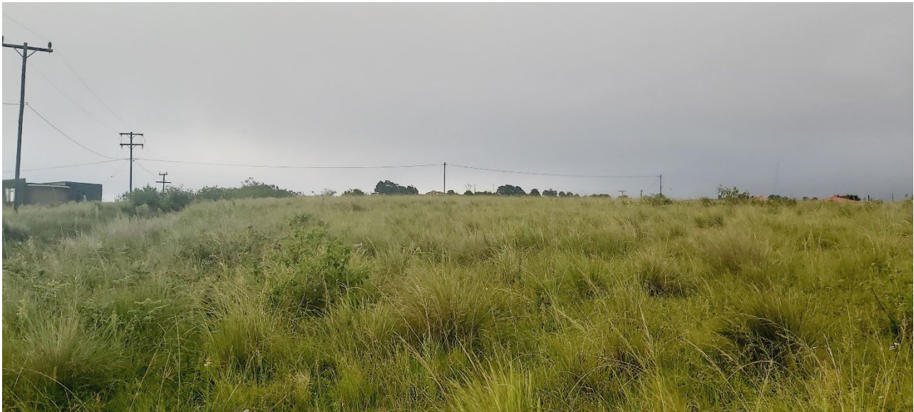
Figure 6. Showing the 22kV powerline traversing the site surrounded by residential dwellings.
